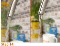
Repeat steps 12 & 13. Run the boil-ing water for 10 minutes, then the filtered water for 10 minutes.
