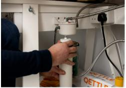
Unscrew the lower section of the filter housing (sump), and empty the residue water into the sink. Place the cartridge into the sink.
